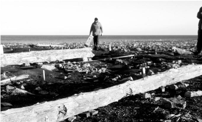
Remaining beams of the wintering cabin, the 'Saved House' and excavation of the cabin's surroundings. In 1997 a life-size reconstruction was built in Amsterdam. Note log-cabin construction closed with ship deck planks, covered with sails (Photo's JJZ).
